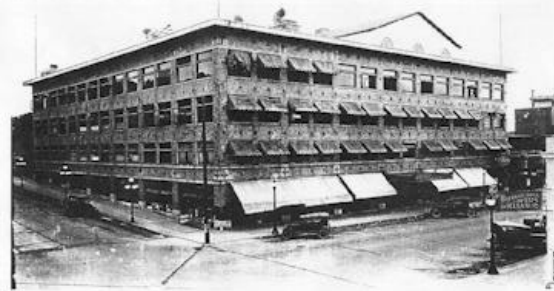
Motor Mart (Commerce Building) 520 Nebraska Street National Register of Historic Places
